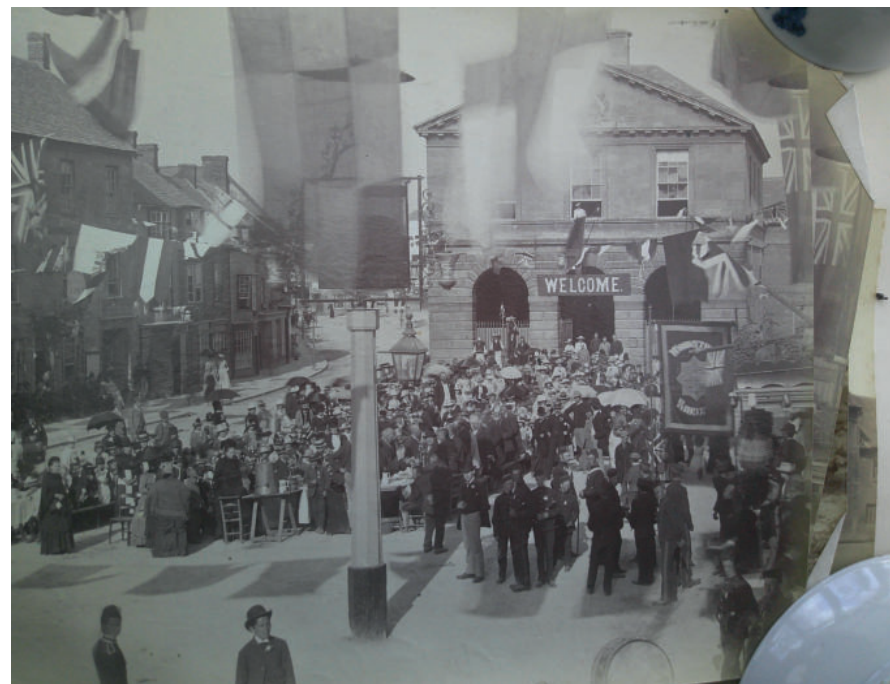
Credit: John Banbury's family photo archive
