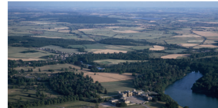
Existing aerial view from Blenheim Palace to the south east
