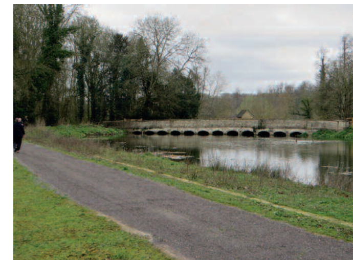
A bridge along the Blenheim Community Path linking Long Hanborough and Bladon
